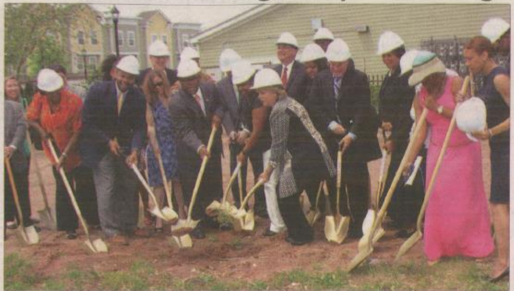
Local, county, state and federal officials attended a groundbreaking on Tuesday, May 12, for the building of the Walter G. Alexander Village, Phase III housing complex, located on Parrow Street in Orange.
